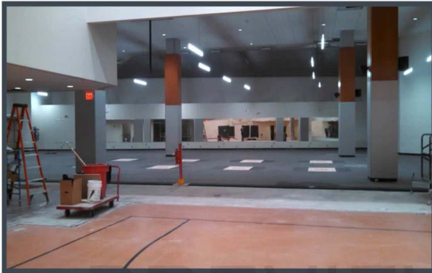
RUBBER UNDERLAYMENT IN WEIGHT ROOM
