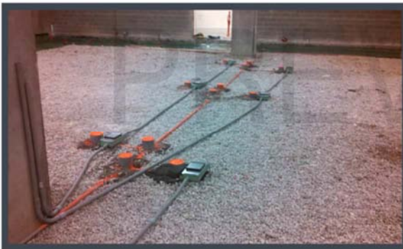
EQUIPMENT & UTILITY LINES UNDER SLAB
