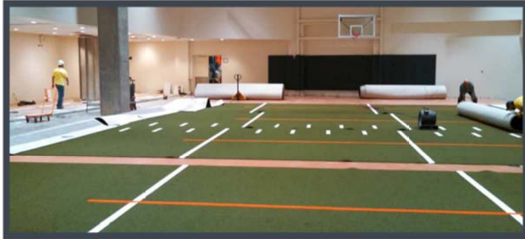
LAYING NEW FIELD TURF
