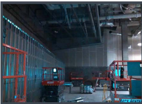
NEW CORRIDOR WALL FRAMING
